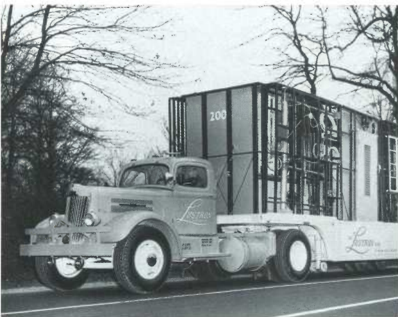
Prefabricated housing was popular in the 1950s. This Lustron truck is delivering a dwelling.
