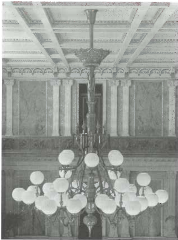
Lighting in historic buildings will be discussed in the conference and in an all-day workshop. The elegant lighting in the Cash Room at the U.S. Treasury can be seen during the lighting workshop. Photo: Gary Griffen
